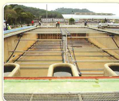
Rectangular Scrapers For Settling Tank
