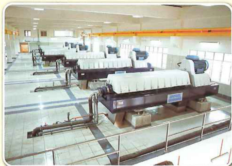
Centrifuge Sludge Decanter
