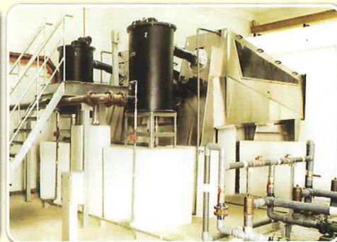
Rotary Drum Thickener
