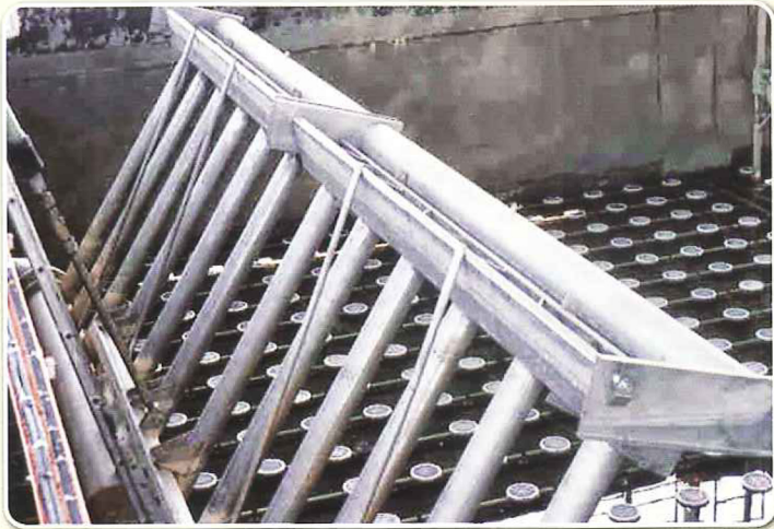
Surface Skimming Decanter
