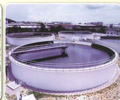
Circular Clarifier Scraper
