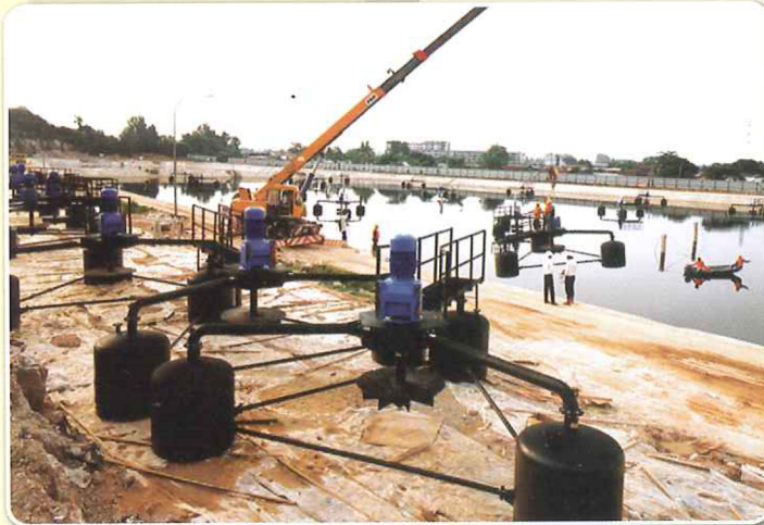
Installation & Upgrading of Oxidation Pond to Aerated Lagoon
