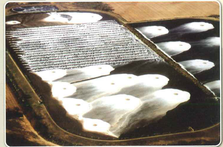
Upgrading Of Pond Using Floating Diffuser System
