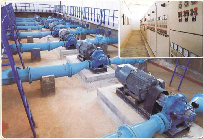
Water Pumping Station
